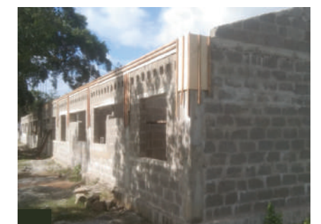
Construction of transit houses at Madu Shrine, Mannar for SLR 400 mn
