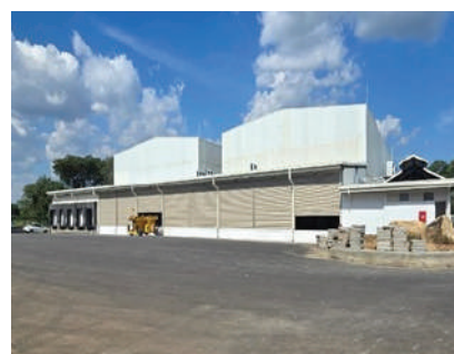
Construction of 5000 MT temperature-controlled warehouse in Dambulla for SLR 300 mn
