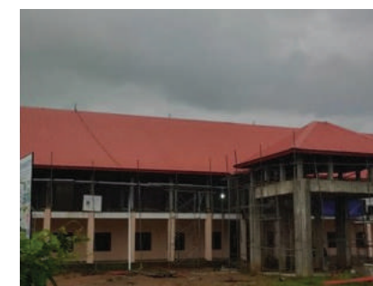
Construction of multi-ethnic tri-lingual school in Polonnaruwa for SLR 369 mn
