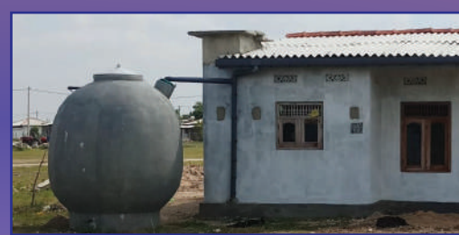
Construction of rainwater harvesting tanks in Jaffna District for SLR 422 million
