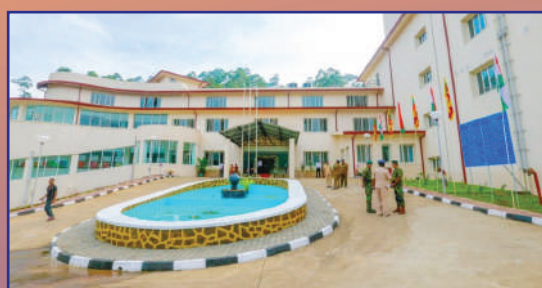
Construction of 150 bed multi- speciality hospital and supply of medical equipment at Dickoya for SLR 1.2 billion
