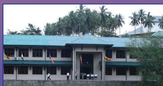
Construction of Kandyan Dancing School at Sri Dalada Maligawa for SLR 145 million
