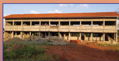
Renovation of 27 schools in the Northern Province for SLR 268 million
